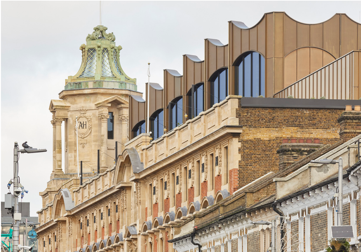
Rooftop extension at the Arding & Hobbs building, London Image courtesy of Stiff + Trevllion/ Wood Awards
